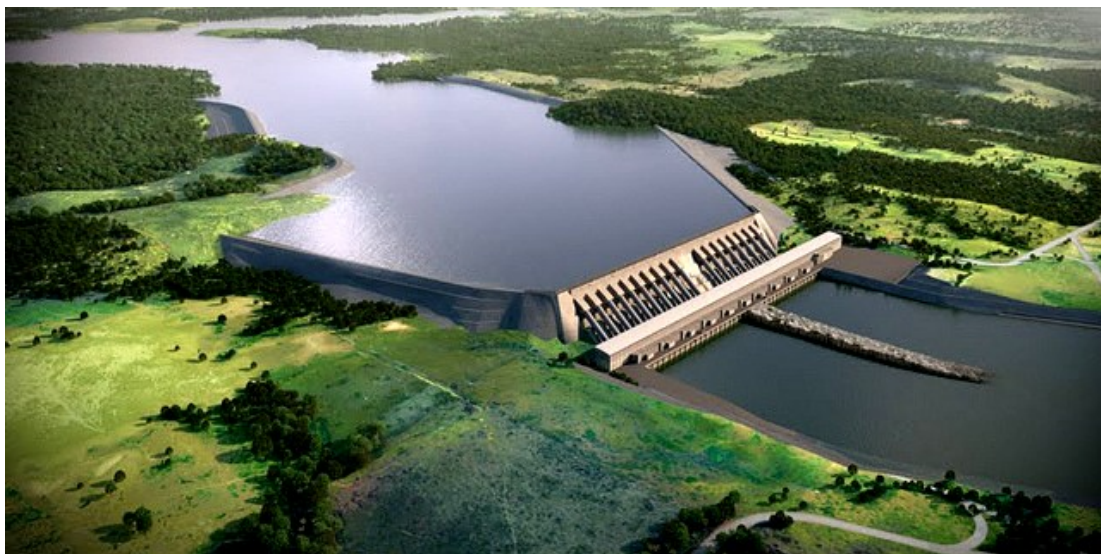
The construction of the Belo Monte Dam in the amazon region of Brazil.
